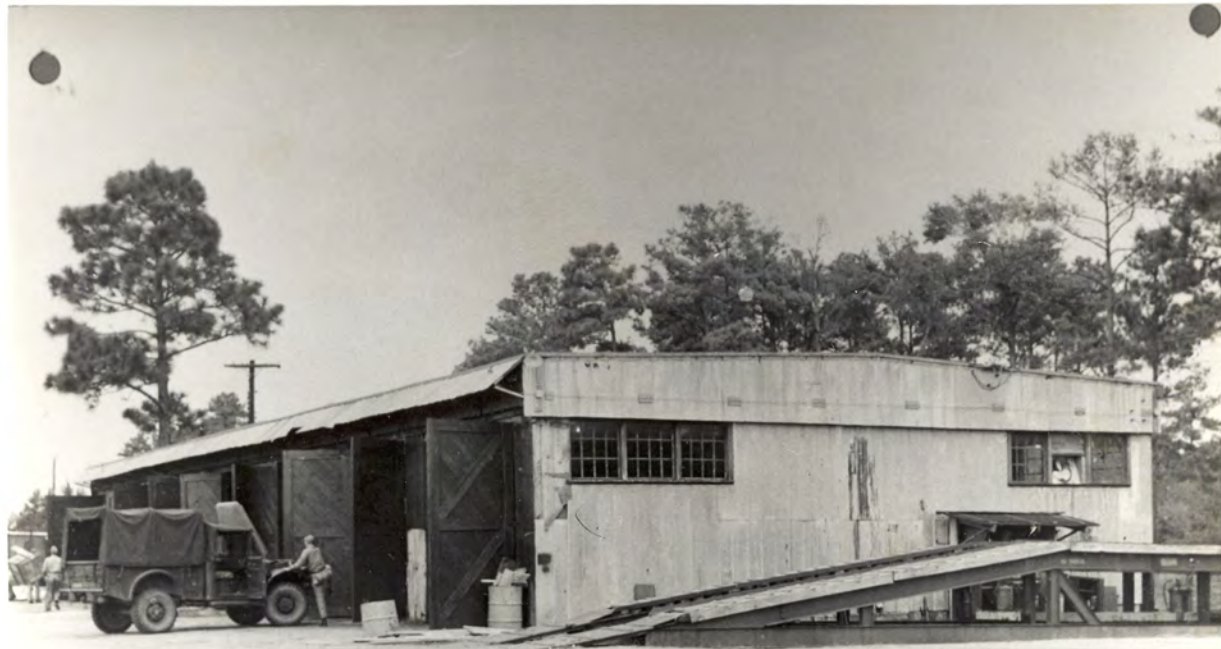
AUTO MAINT. SHOP Bldg. #T-414 Front View Size - 48'x112' Area - 5,376 SF Cooling - None Heating - None Com. Detel - 1942 (WW II) Est. Value - $3,225.60
