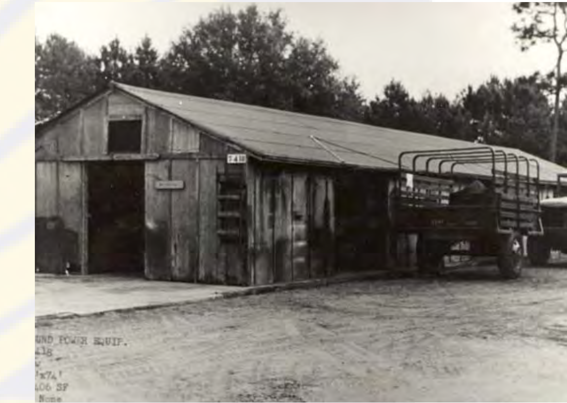
Ground Power Equipment
