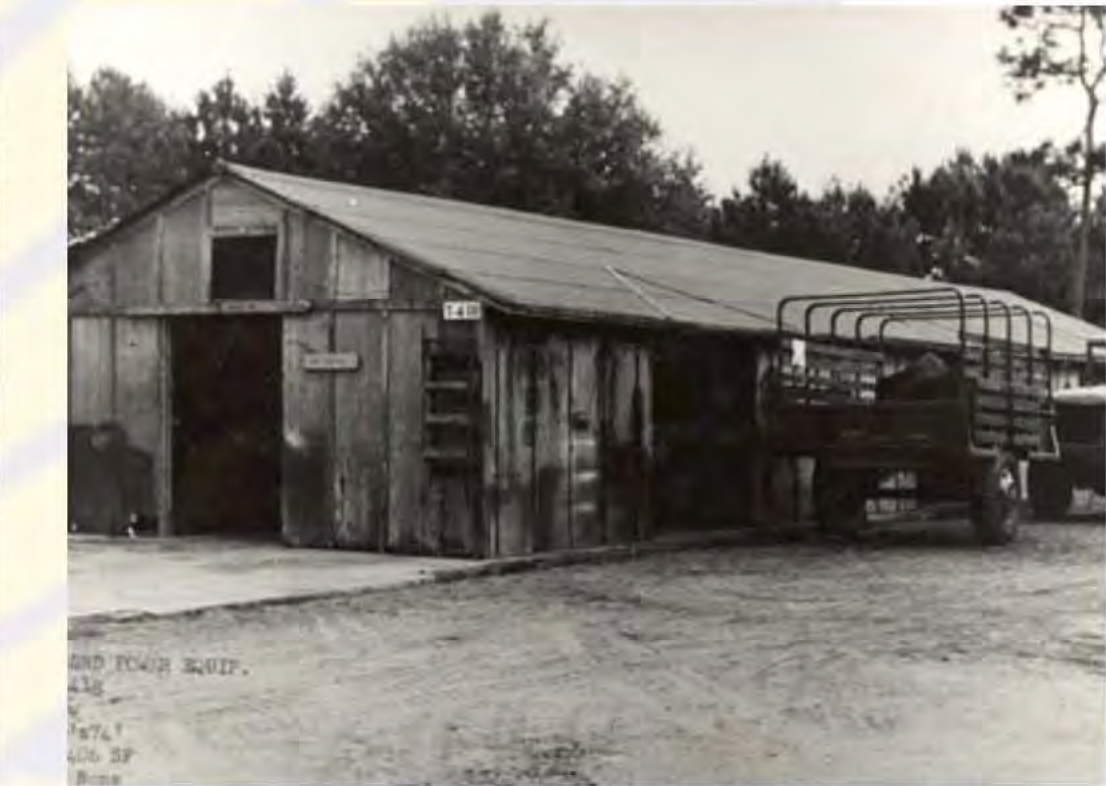
Ground Power Equipment
