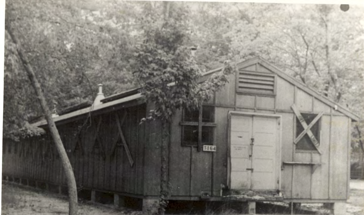
DORM., AIRMAN Bldg. #T-164 Front View Size - 20' x 100' Area - 2,000 SF Cooling - None Heating - None Completed - 1942 (WW II) Est. No. 1164
